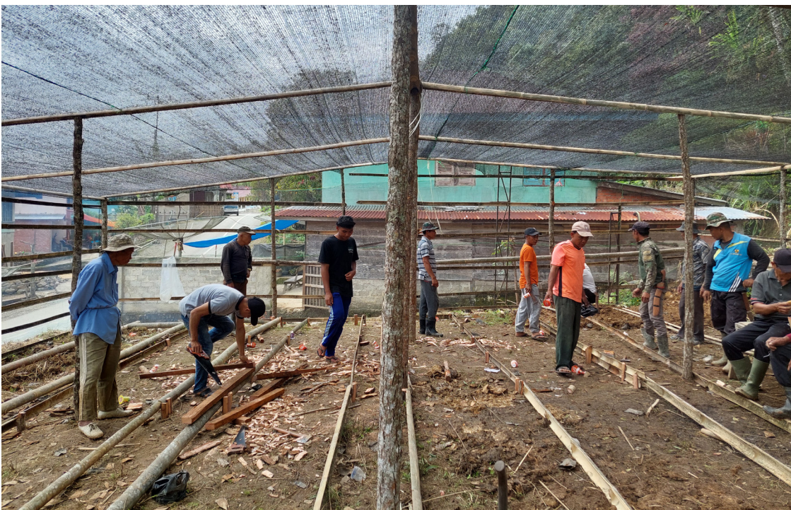
The process of building seedling house in Pungut Hilir Village
